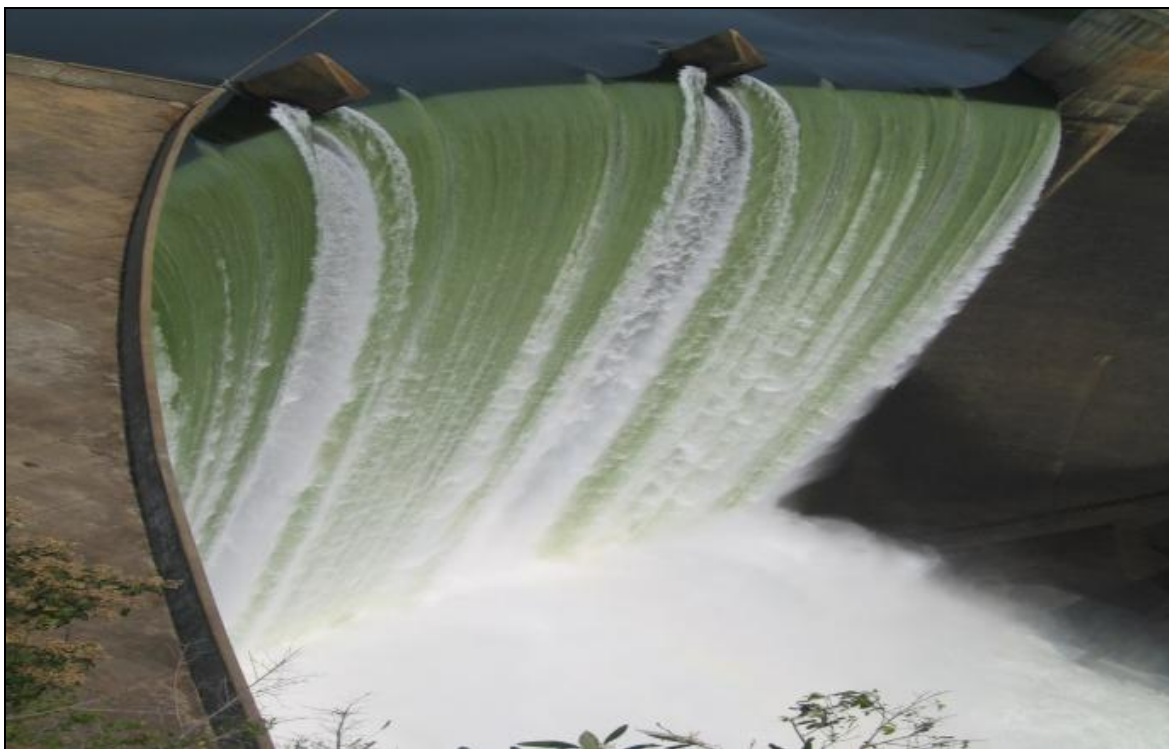
Figure 9: Cambambe hydro electric power station
