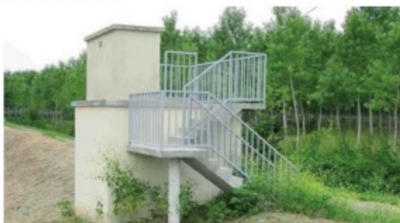
d. Elevated battery energy storage system
