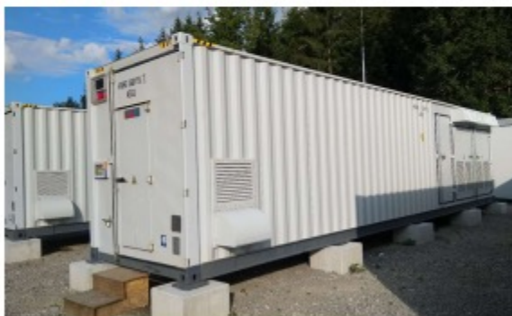
d. Elevated battery energy storage system
